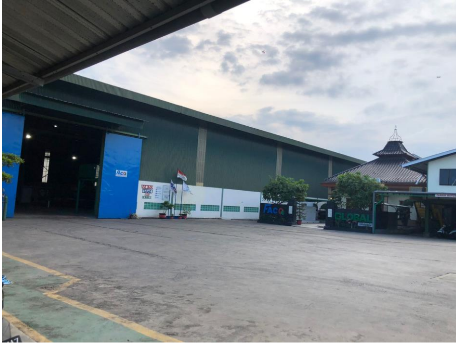
Gambar 2.1 Gedung PT. Faco Global Engineering
